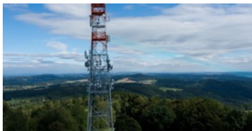
Power cellular towers
